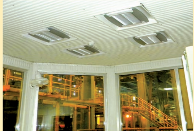
Control Cabin False Ceiling
