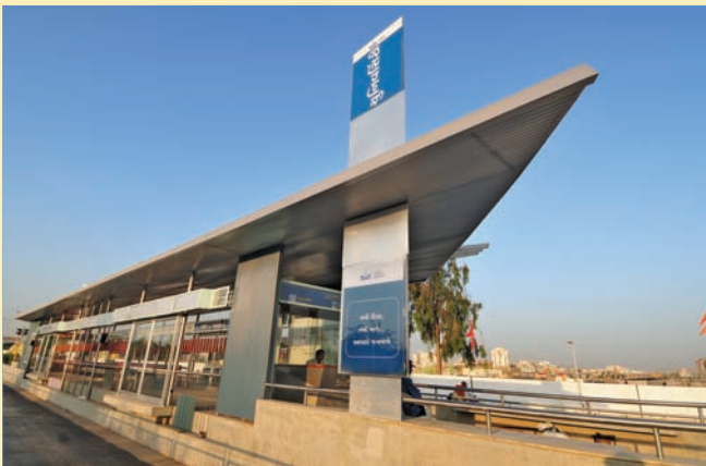
Bus Stop False Ceiling
