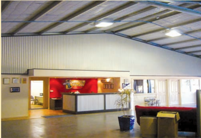
Canteen Interior Wall Panel
